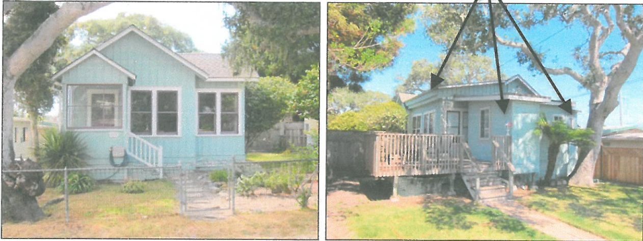
Figures 1 and 2. Left image shows the front (west) elevation of the house. The porch and stairs were installed circa-1940s. Right image shows the rear (east) elevation with additions (arrows).
